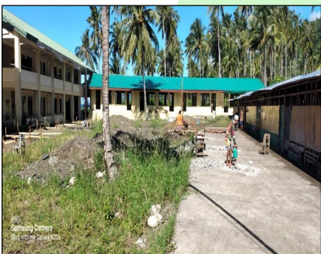
Improvement of School Building-Sitio Lilinaban Elementary School (Barangay Tabayon)
