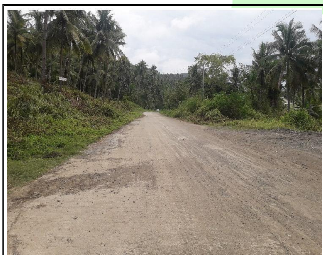
Road Repair (Barangays Caburan Big)
