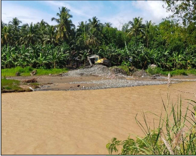
Desilting of Culaman River (Barangay Culaman)
