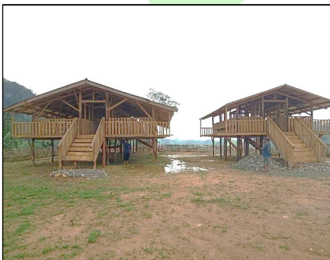
Two (2) units-Goat Multiplier Farm House (Barangay Demoloc)
