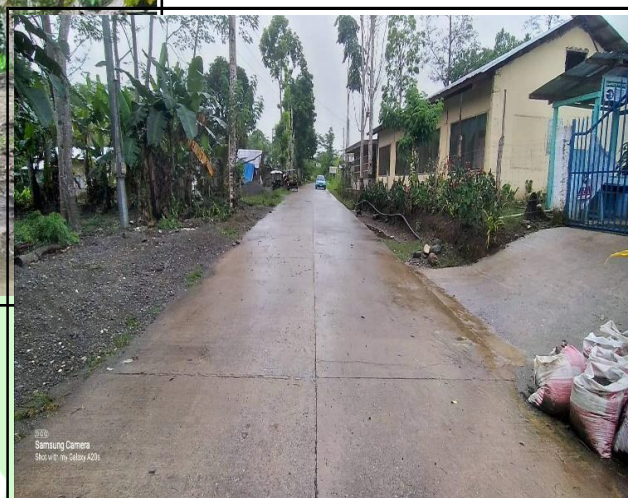
Road Concreting (Barangay Datu Danwata)
