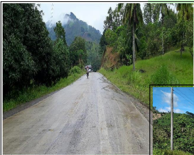
Rehabilitation/Concreting (Demoloc-Kilalag-Pinalpalan Road Phase I)
