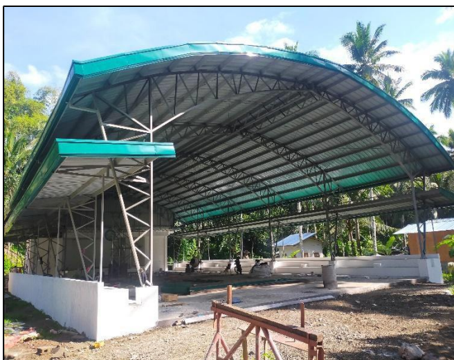
Covered Court with Stage and Toilet @NHS (Barangay Talogoy)
