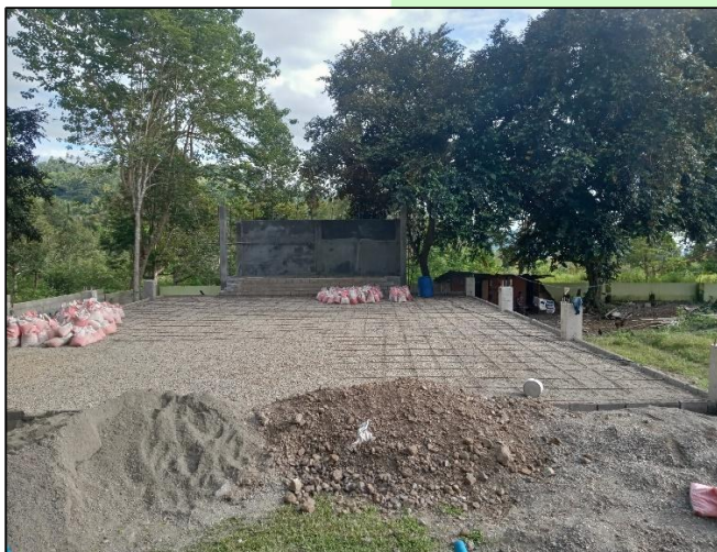
Mini-Gym/Covered Court w/ Stage @ Elem. School (Barangay Lais)
