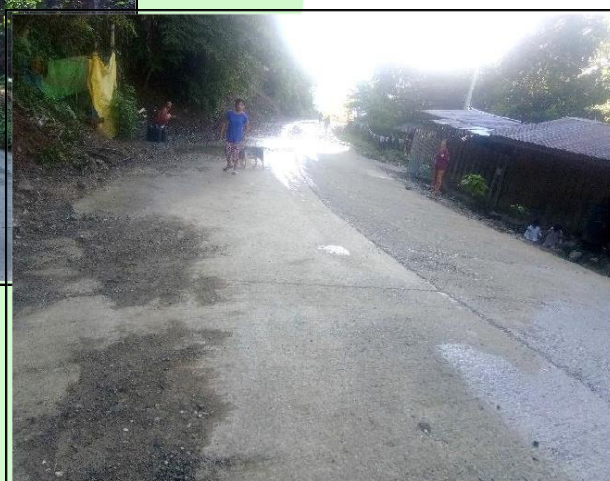
Road Construction Mahayahay-Mote-Pinalpalan Proper Brgy. Road (Barangay Kilalag)
