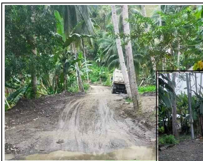
Gravelling of Road (Barangay Pinalpalan)
