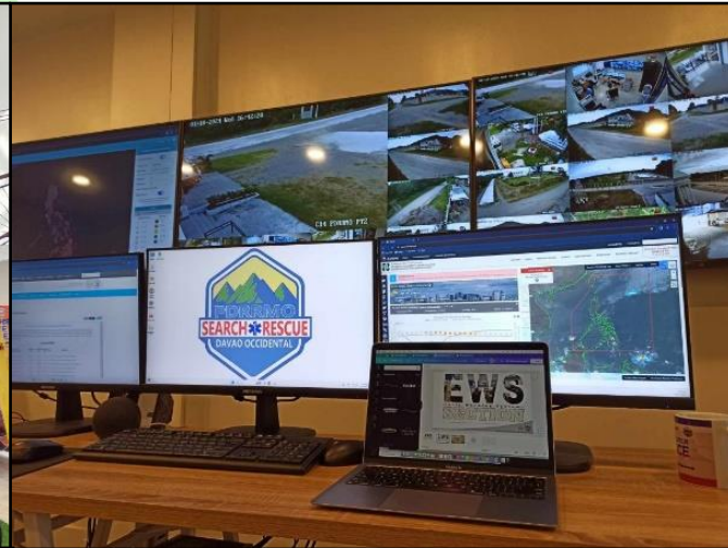
PROCURE AND INSTALL EQUIPMENT AND FACILITIES FOR EARLY WARNING SYSTEMS
