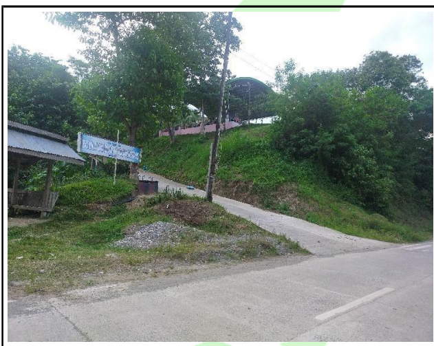
Road Concreting @ NHS (Barangay Bolila)
