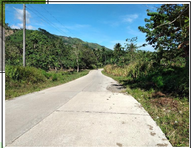
Rehabilitation/Concreting (Demoloc-Guisok-Sarangani Road Phase I)
