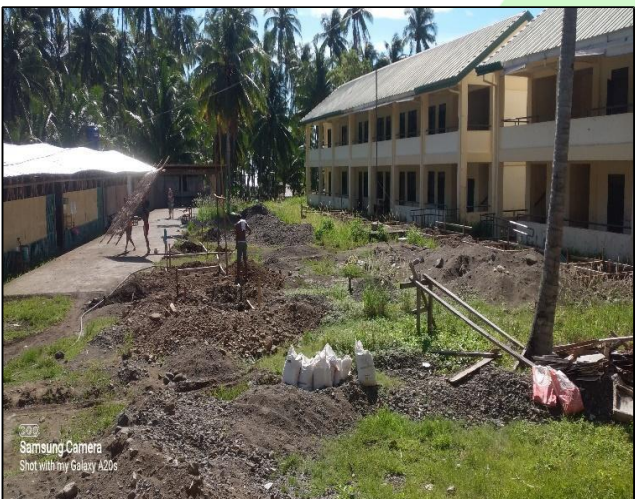
Covered Court with Stage & Toilet @NHS (Barangay Tabayon)
